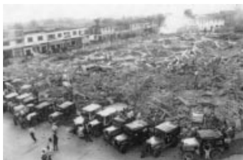
Figure 5 Destruction of the central park of Calarcá.
